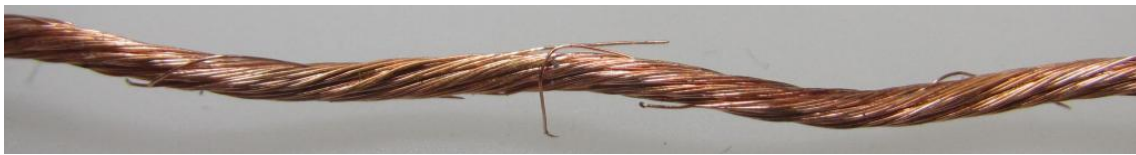
Close-up of the conductor rope
